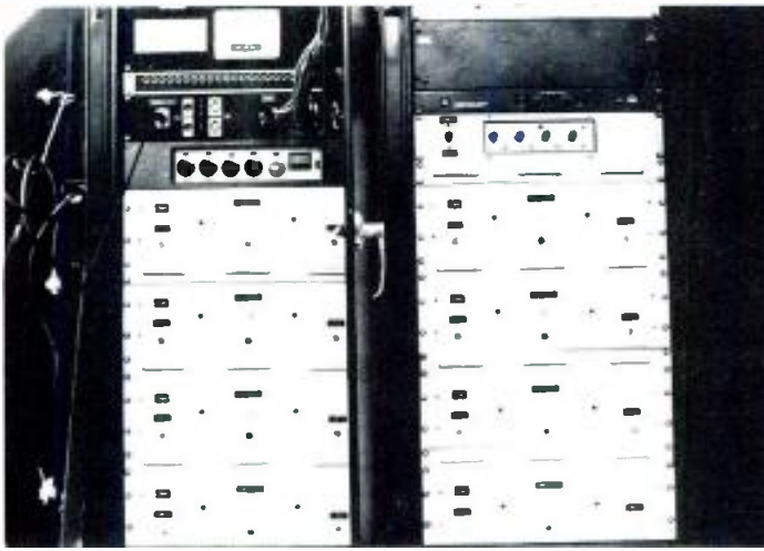
The two sound racks are located on the speaker tower trailer at truck bed level, with a matching pair on the other truck, each speaker unit operating independently. On the left is a mic mixer, patch and connection panels, a line level a.c. meter, the master switch panel, and 4 amplifiers. The right rack holds 4 amps, the complimiter, the crossover network, equalizer, and notch filter.
